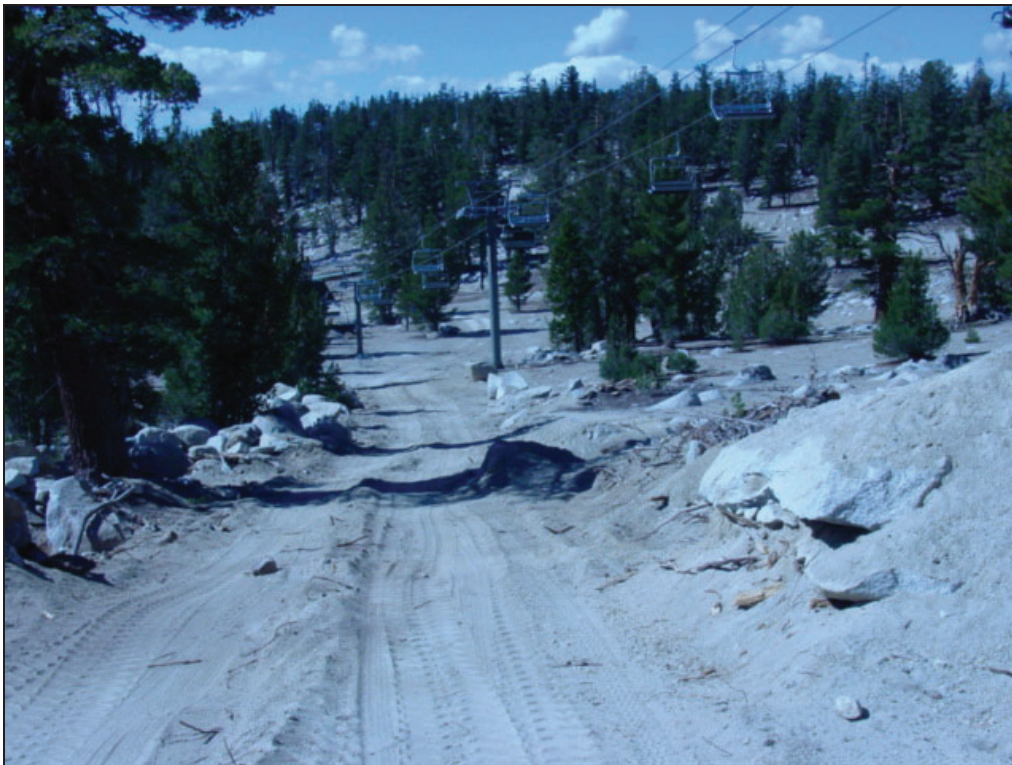
Photo 3: Easy Street Segment 2, pre-treatment conditions.
