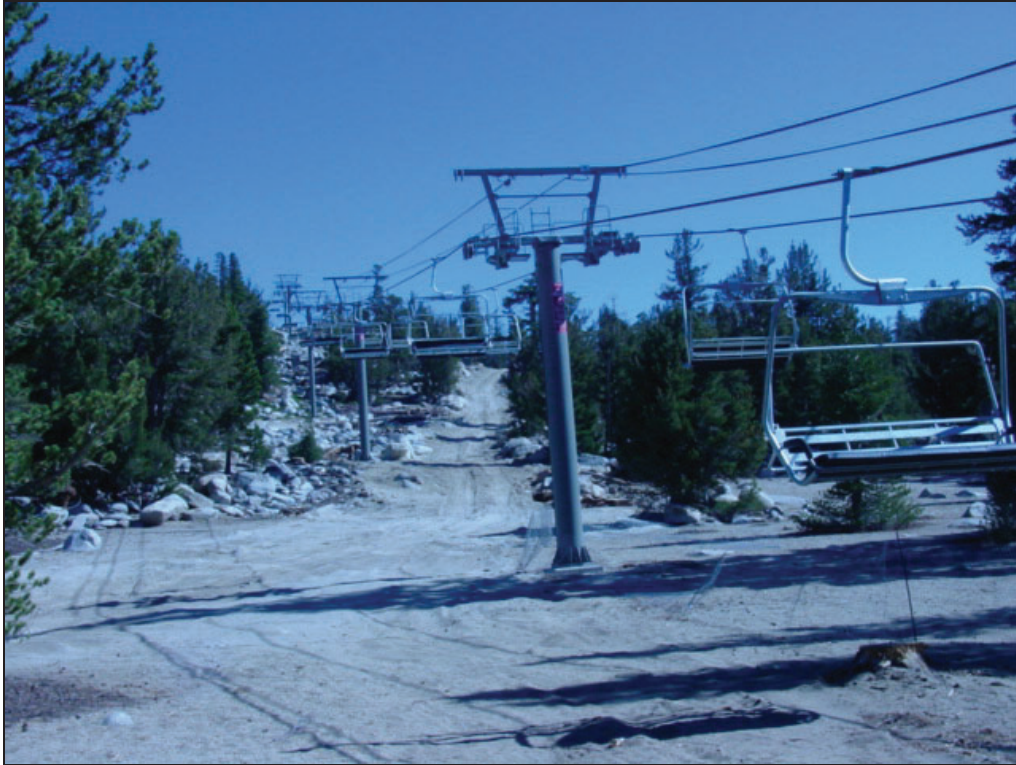
Photo 4: Easy Street Segment 3, pre-treatment conditions.
